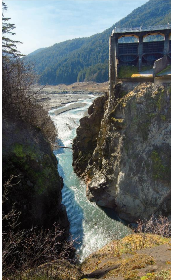
Goodbye to a large dam. Elwha River passing through the remains of Glines Canyon Dam on 21 February 2015. The former Lake Mills can be seen in the background.
